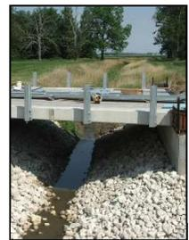
Figure 2: Slab bridge
