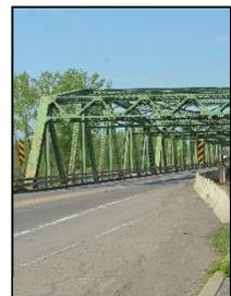
Figure 3: Truss bridge
