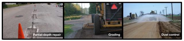
Figure 6: Examples of capital preventive maintenance treatments, cont'd—(from left) concrete road prepared for partial-depth repair, gravel road undergoing maintenance grading, and gravel road receiving dust control application (dust control photo courtesy of Weld County, Colorado, weldgov.com).
