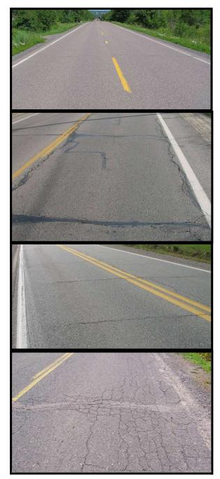
Figure 1: *Top image, right*– PASER 8 road that is considered "good" by the TAMC exhibit only minor defects. *Second image, right*– PASER 5 road that is considered "fair" by the TAMC. Exhibiting structural soundness but could benefit from CPM. *Third image, right*– PASER 6 road that is considered "fair" by the TAMC. *Bottom image, right*– PASER 2 road that is considered "foor" by the TAMC exhibiting significant structural distress.
