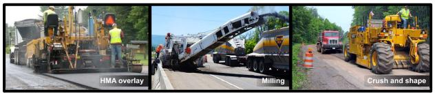
Figure 4: Examples of structural improvement treatments—(from left) HMA overlay on an unmilled pavement, milling asphalt pavement, and pulverization of a road during a crush-and-shape project.
