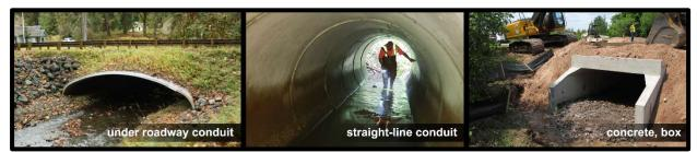
Figure C-2: Examples of culverts. Culverts allow water to pass under the roadway (left), they are straight-line conduits with no intermediate drainage structures (middle), and they come in various materials (left: metal; middle and right: concrete) and shapes (left: arch; middle: round; right: box).
