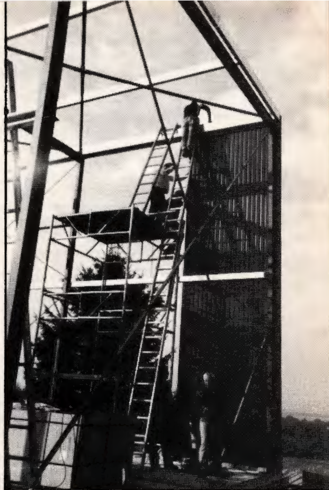
The insulation goes up on a single court being built at a NATO Air Base on the German/Dutch border. (Above).
