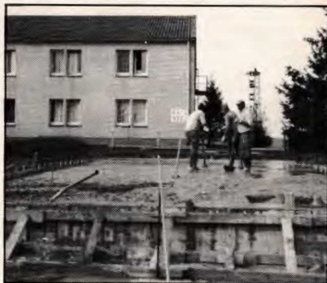
The foundation being poured on a single racquetball court going into an isolated missile site near Luxembourg.
