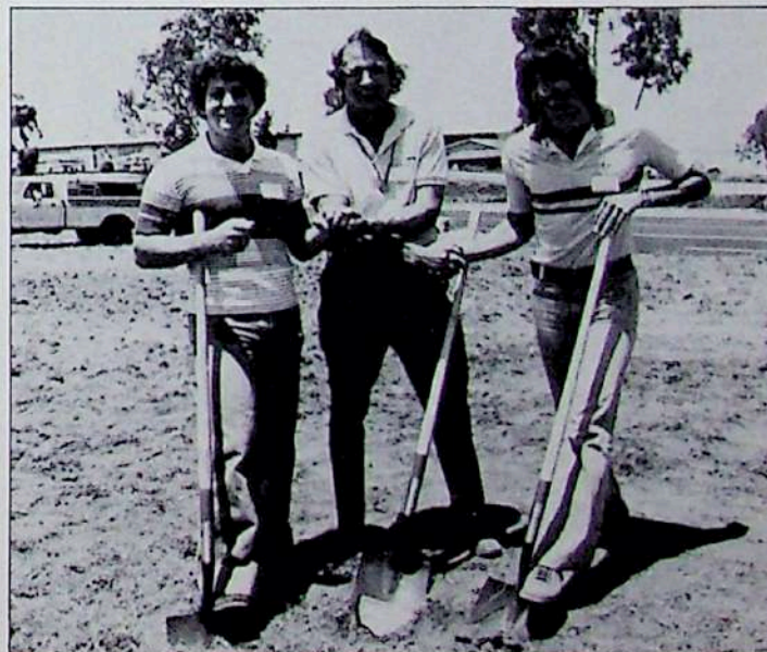
Ektelon President Bud Held gets a helping hand from two top Ektelon player professionals during recent groundbreaking ceremonies for Ektelon's new 64,000-square-foot manufacturing plant in San Diego. Mike Yellen, at left, and Jerry Hilecher, at right, help Held toss the first few spadefuls of dirt during a groundbreaking.
