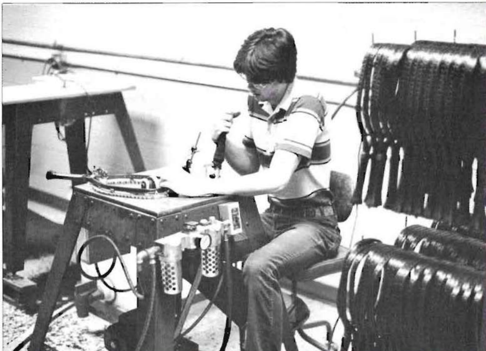
Hand-drilling an injection molded racquet.
