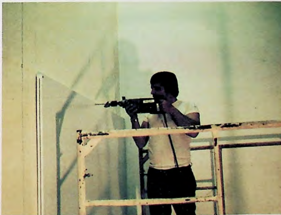
Installation of panels were made to remedy a damaged front wall on one of the courts at the Northwest Suburban YMCA. The subsequent success of this job led to use of the panels in the additional courts.
