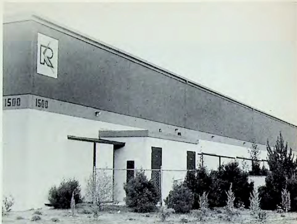
The utilitarian appearance of the Pay 'N Play courts blends with the other buildings in an Anaheim industrial park.
