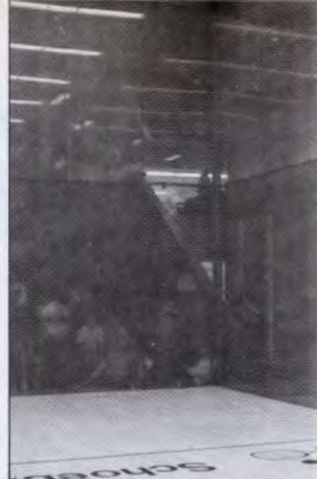
One problem that still remains is more clearly defining the juncture of two Twin-Vue walls. From inside the court, you're looking at the front and side wall right corner, which does lack clear definition.
