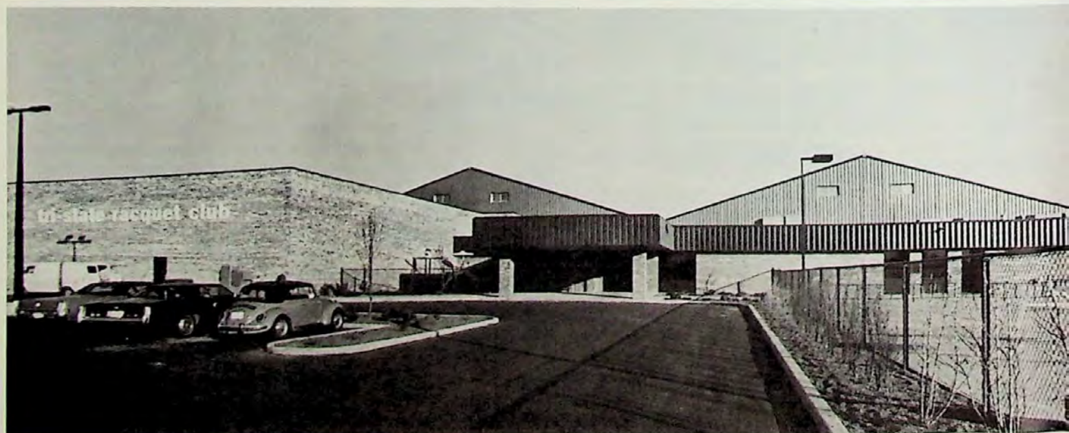
The new Tri-State Racquet Club, Evansville, Ind., recently was opened including seven air conditioned racquetball/handball courts, eight air conditioned tennis courts, eight outdoor courts and outdoor pool. It is the only club of its kind in southern Indiana, Illinois and Kentucky.
