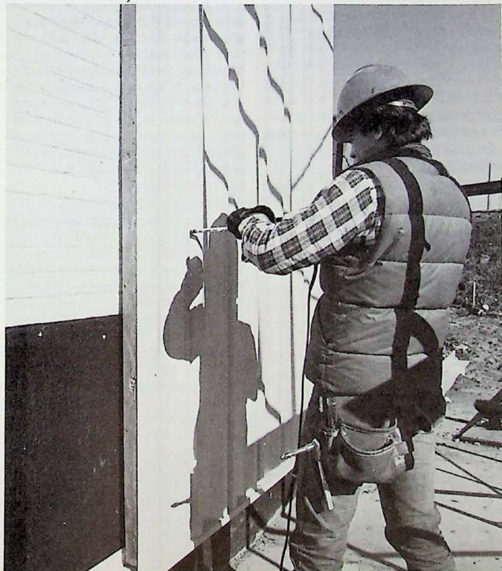
Retrofitting buildings with pre-engineered steel is a relatively simple process that provides a cost-efficient and energy-efficient alternative to new construction. Photo courtesy of Star Manufacturing Co.
