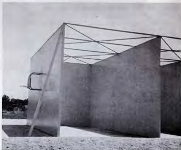
Angle view shows how outside side walls can be utilized for basketball, tennis practice, or one-wall play. The multi-purpose use of this installation "sold" Detroit Parks and Recreation Department.
