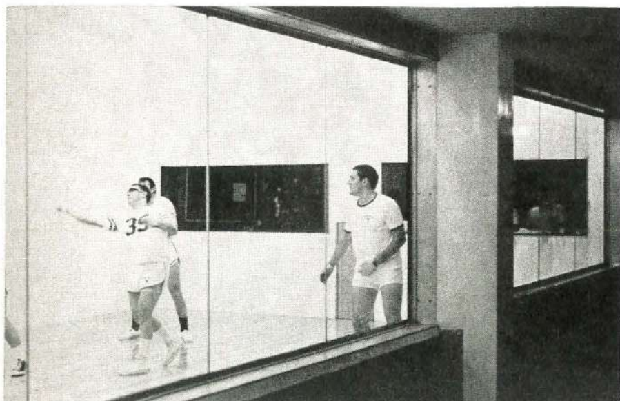
CHAMPIONSHIP COURT AT CHARLOTTE . . . Glass in both back wall and left side wall will afford seating for upwards of 150 during South USHA divisional. Portable bleachers will be set up behind the glass. Note that mullions have been eliminated giving clear view to all. There is also viewing area from balcony above back wall. Other three courts have glass in back walls.
