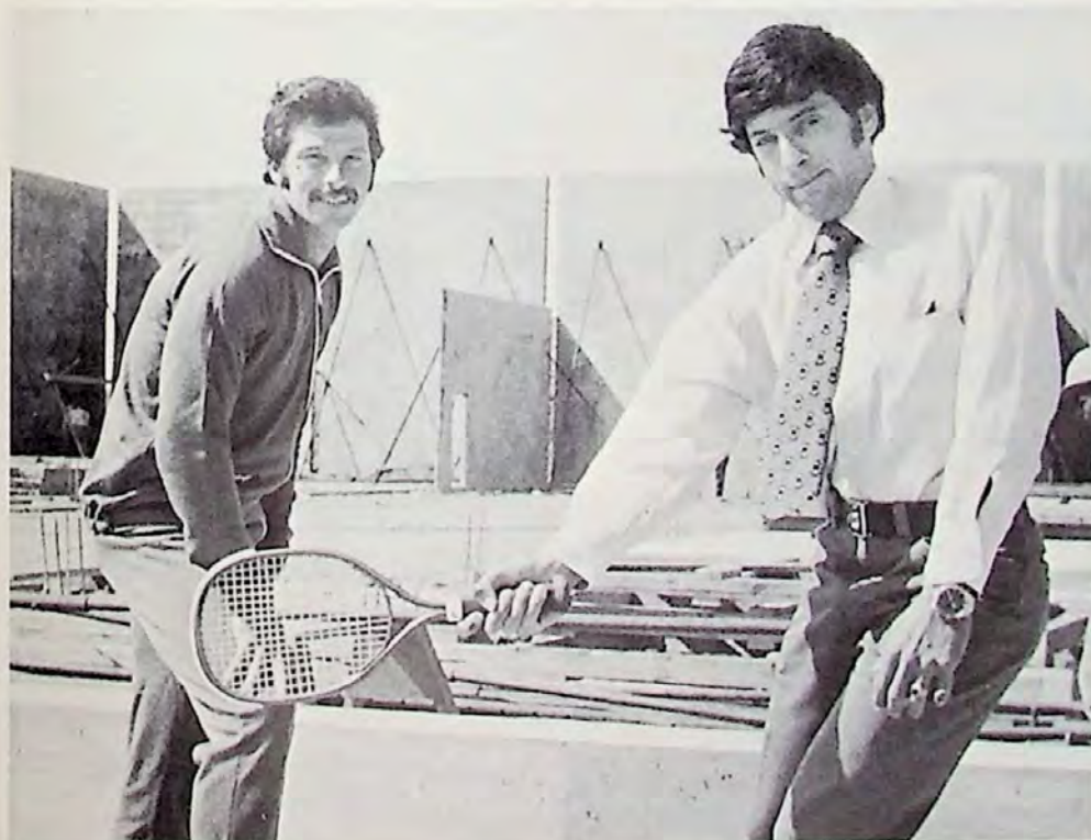
Walls of the Schoeber's club on the way up with tilt-up concrete construction. In the foreground are club manager Howard Wasserteil (r.) and exercise physiologist Ben Friedlander.
