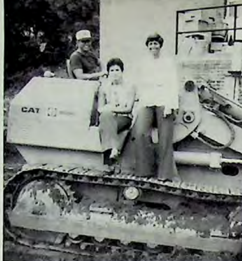
CAT DRIVER gets help from Pamela Hanes and Nancy Gingerich during construction of the club and (lower left), a Bentley auto graces the front lawn at a much later stage of construction.
