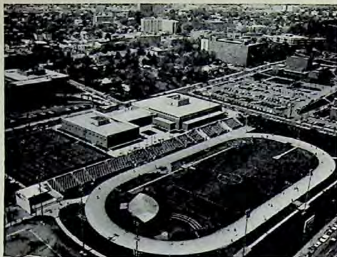
NEW PHYSICAL EDUCATION BUILDING — The NPA Championships will be held May 4-7 in the new P.E. Building on the University of Tennessee's Knoxville Campus. The building is bordered by the Tom Black Track, which features a Tartan covered surface, tennis courts and intramural fields.
