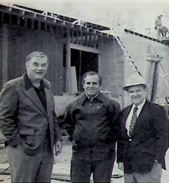
From left to right Dick Peters, local developer, Herb Widensol, general contractor, and Charles Spaulding, president of the Spaulding Racquetball Clubs, Inc., in front of the new Spaulding Club as it neared completion at 2300 W. 6th St. in Lawrence, KS.
