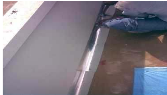
Flashing at Ridges Valleys & Wall joints
