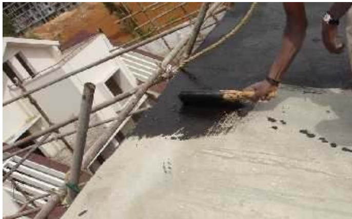
Surface Cleaning by applying Bituminous Primer
