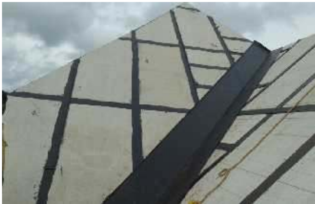
Surface Cleaning by applying Bituminous Primer
