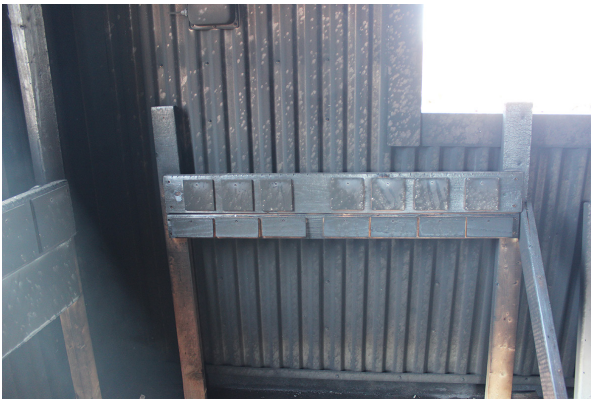
Figure 4 Photograph showing the soot covered down to about 2 feet.
