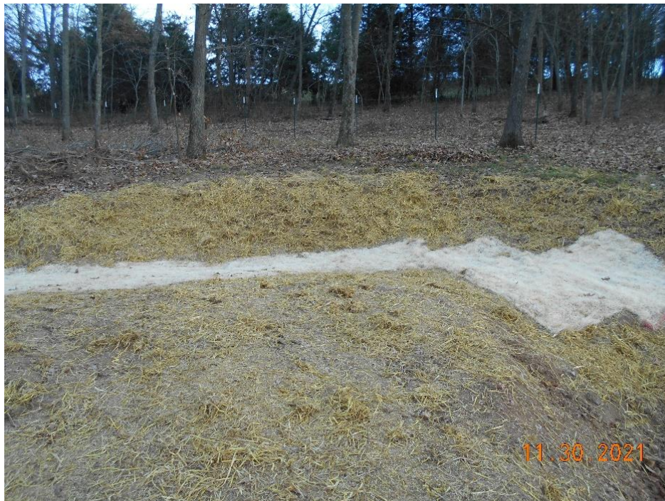
Erosion Control Blanket on the emergency spillway.
