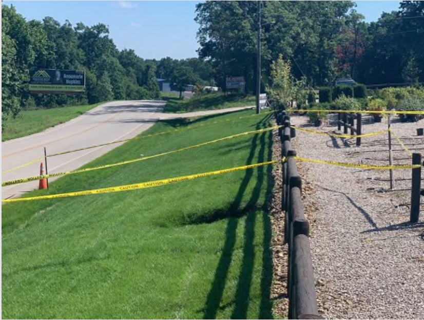
A sinkhole discovered Wednesday, August 17, 2022, in front of Doctor's Landscaping in the Sunrise Beach area of Lake of the Ozarks.
