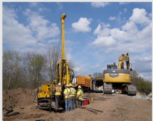
Bridge construction on Highway 163 near Columbia, Mo.
