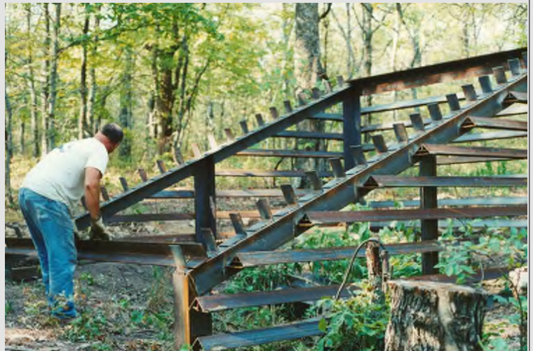
Billy building a bat grid gate (2001)
