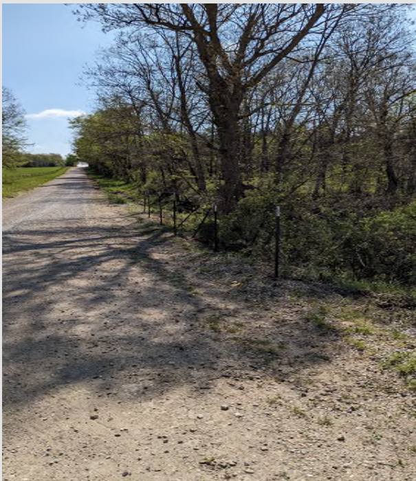
Cleaned and ready for the new fence
