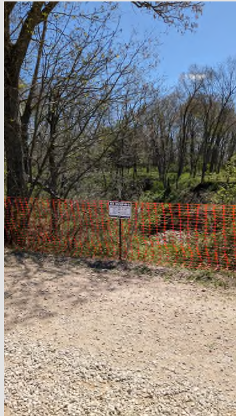
New fence and sign installed
