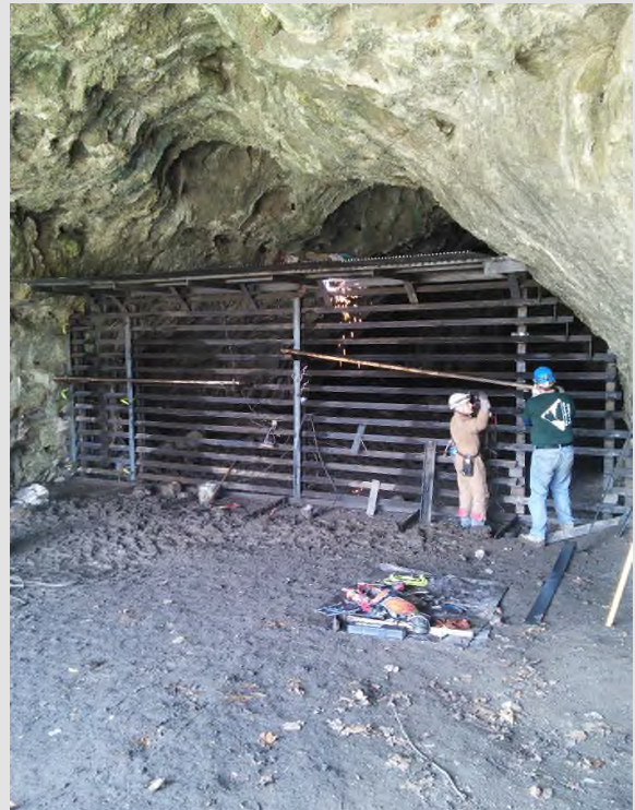
Above and left: building the new gate
