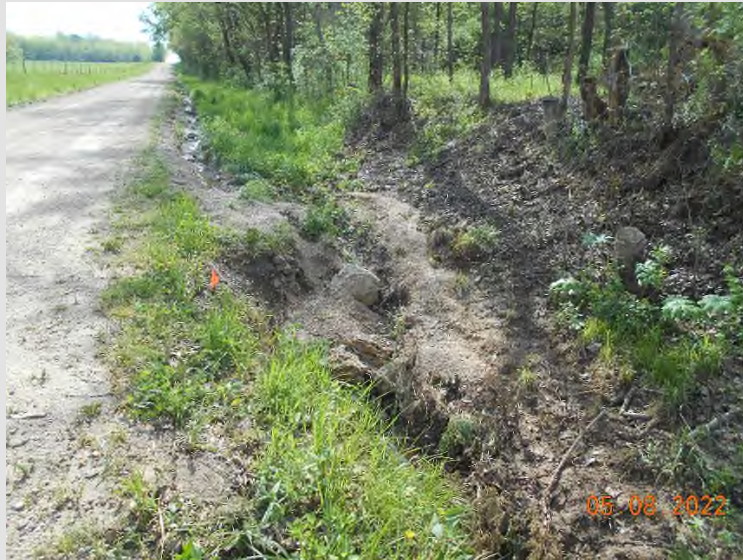
Extensive erosion along Lancaster Road near the sinkhole.
