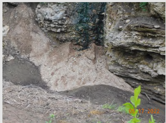
Gravel deposited below the waterfall. I estimate that the amount would fill about 4 dump trucks.
