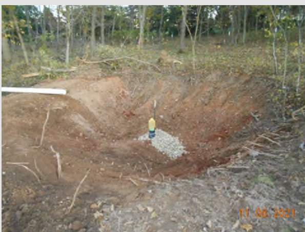
Photo taken in November 2021 during construction of the catch basin. Note: A standpipe drain would allow the trapped water to drain out via the buried culvert and prevent any additional erosion from occurring in the back of the sinkhole.
