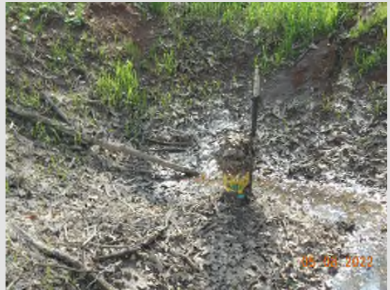
The catch basin on May 8, after the water level had receded. Notice the debris on top of the water intake.
