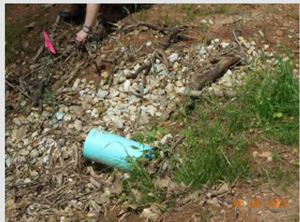
Photo taken in November 2021 during construction of the catch basin. Note: A standpipe drain would allow the trapped water to drain out via the buried culvert and prevent any additional erosion from occurring in the back of the sinkhole.
