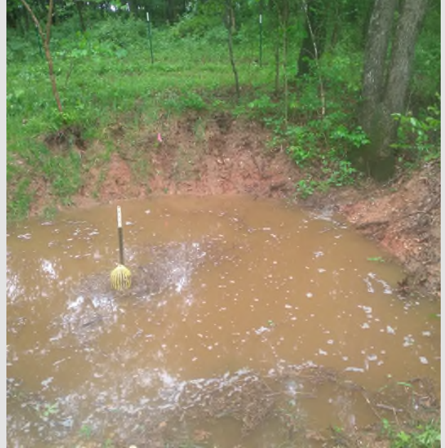
Photo taken on May 21, of a nearly full catch basin. Notice the top of the yellow water intake next to the fence post. Ken said that he could see the water entering the water intake.
