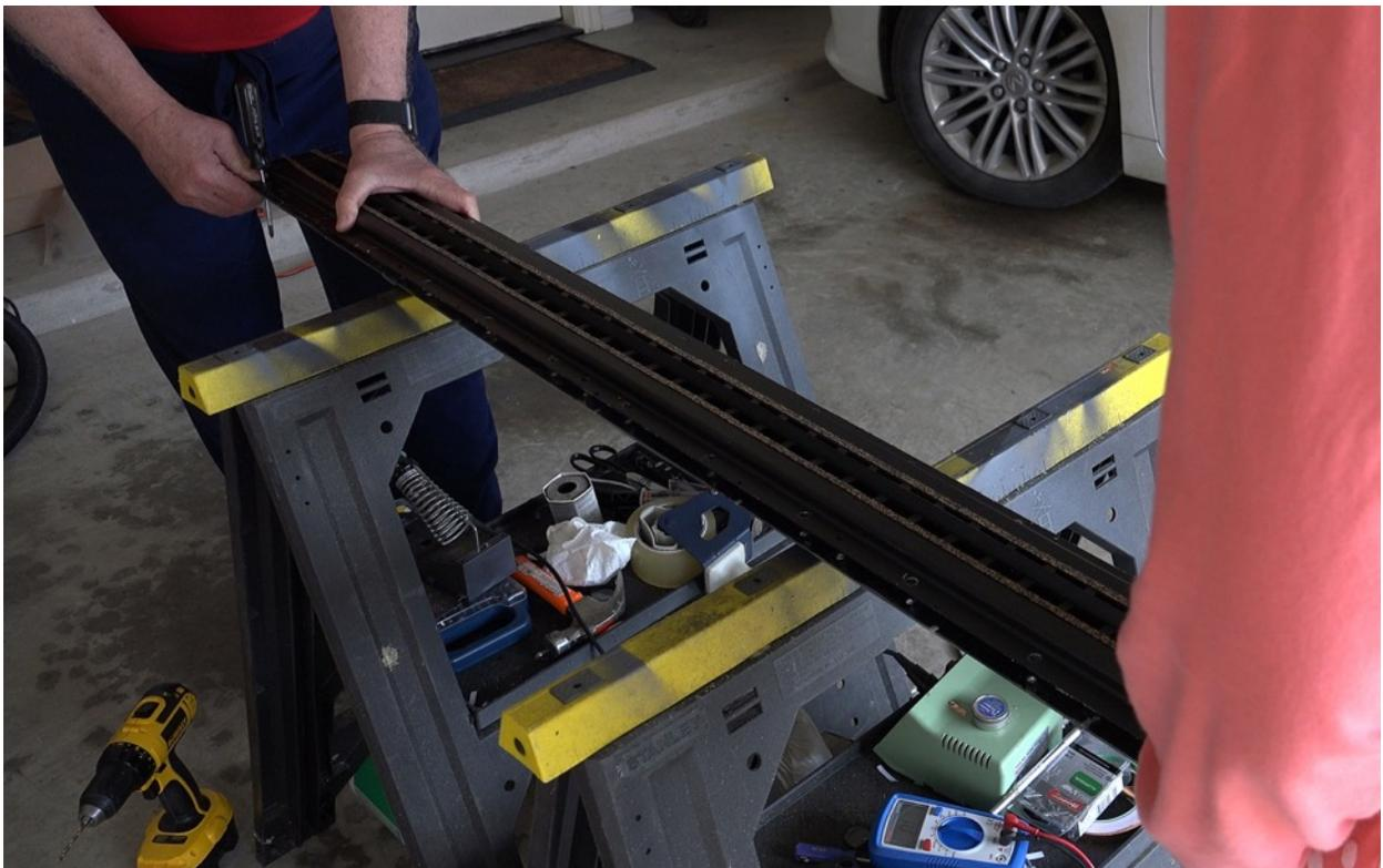
With some help from my wife we pressed the top and bottom halves together and I installed one rivet at each end to secure. This was not easily done since the powerful magnets in each half of the clamshell are set to repel the two halves! But, once the rivets were in I could install some clamps on either side to make sure the halves were firmly squeezed together before installing the rest of the rivets.
