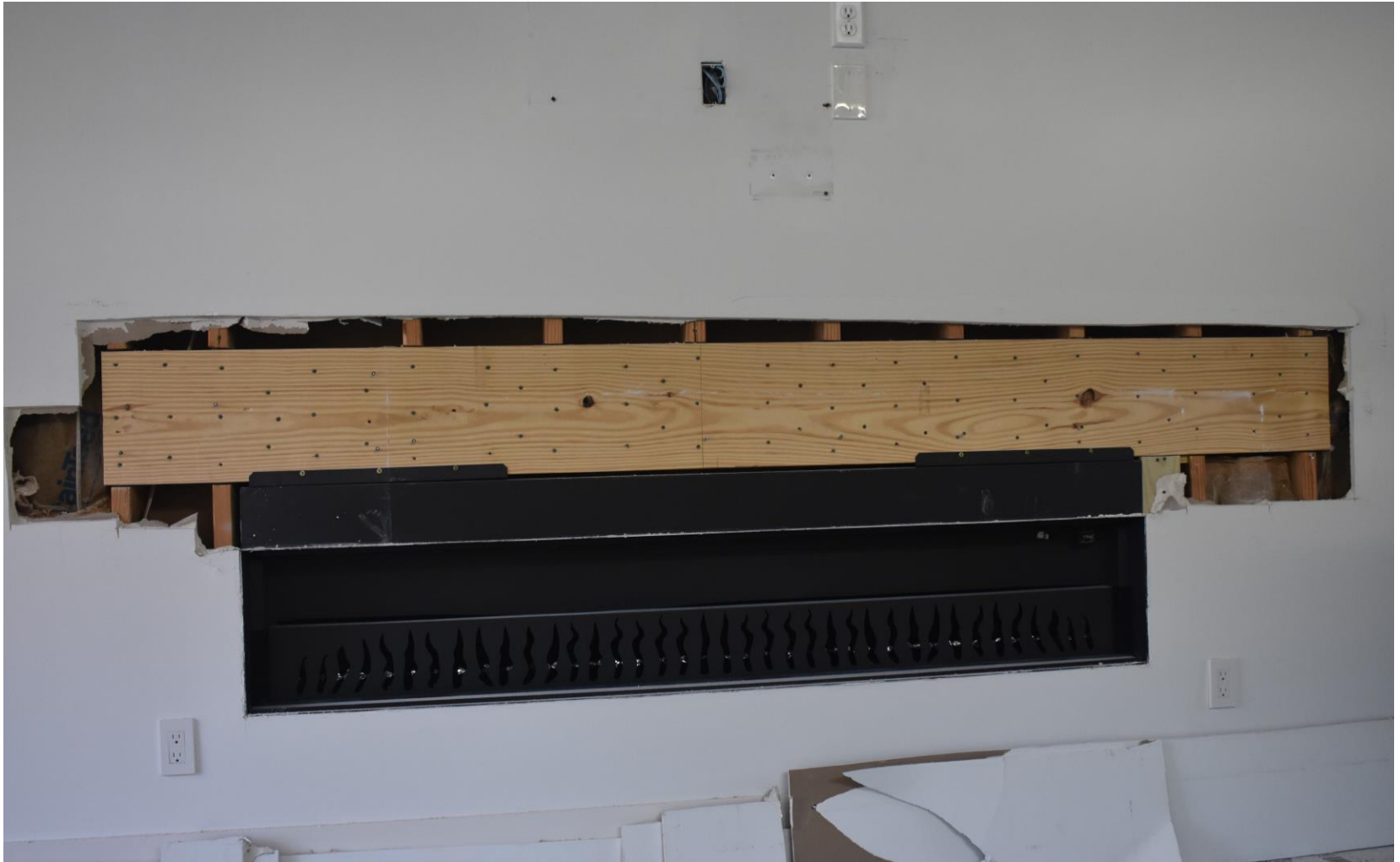
Initial view of the fireplace insert with the header exposed.
