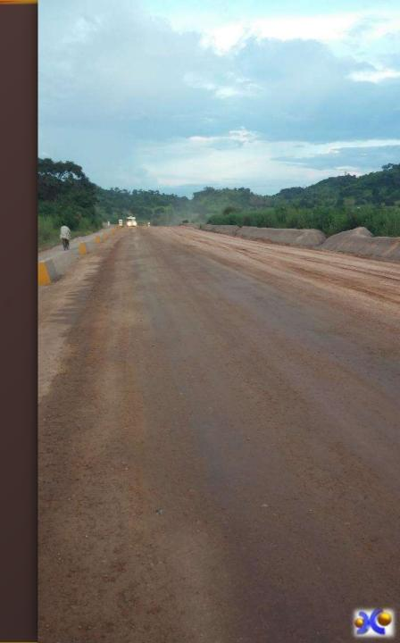
ECOBOND **DURAGRAV** IS A STABILIZED GRAVEL ROAD WEARING COURSE, WHICH IS SURFACED AND MAINTAINED WITH A SPRAY-ON TREATMENT
