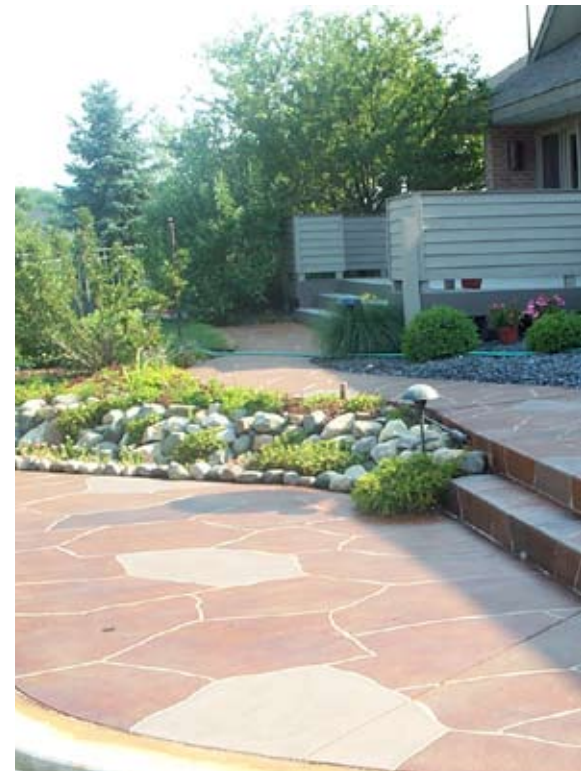
▲ Concrete Resurrection Water Reducible Concentrate (WRC) Stains offer more color choices and a more predictable result. Consider the environment and traffic levels to determine which application will work best. Your decorative concrete professional is trained to answer your questions and to help you make the right choice
