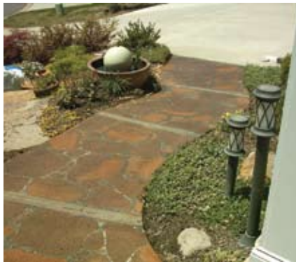
▲ Reactive Acid Chemical Stains (RAC) are ideal for outdoor applications. While permanently changing the color, they allow the natural patterns and character in the concrete to show through
