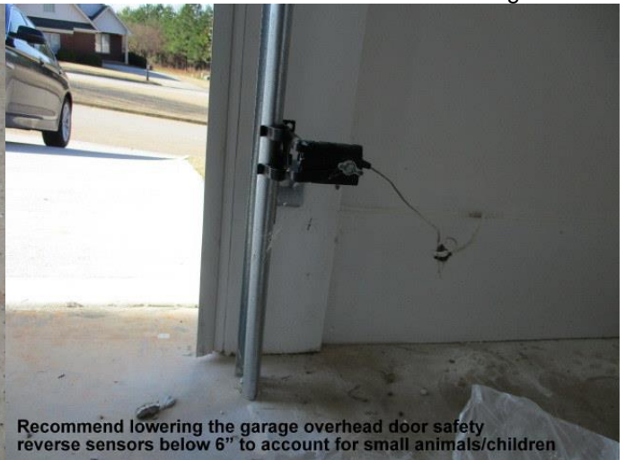
Garage interior door does not seal properly when closed
