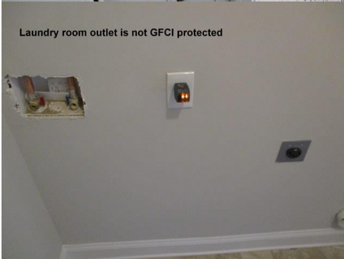
Laundry room washer supply valve housing frame is missing
