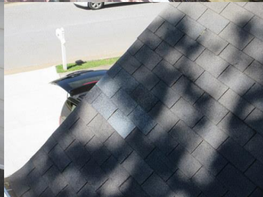
Patches found at the back and front sides of the roof
