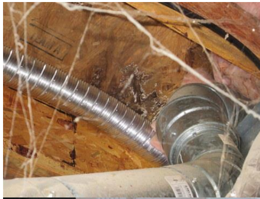
Daylight can be seen in the garage recommend sealing
