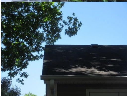
Recommend caulking at the exterior and gas line
