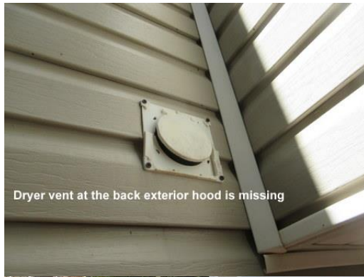
Dryer vent at the back exterior hood is missing
