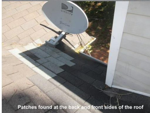
Shingle tabs are missing from the roof and felt is exposed recommend roof replacement
