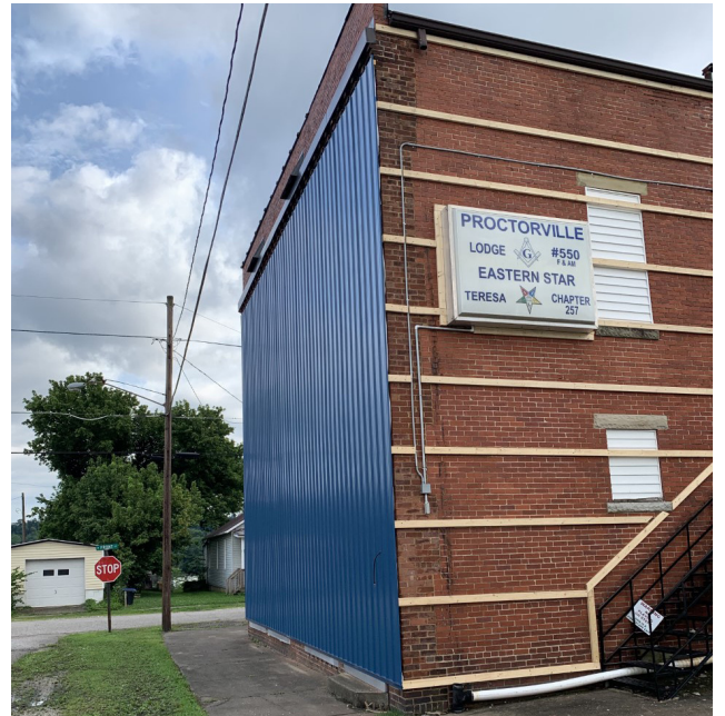
Lodge Building undergoing our exterior remodeling program
