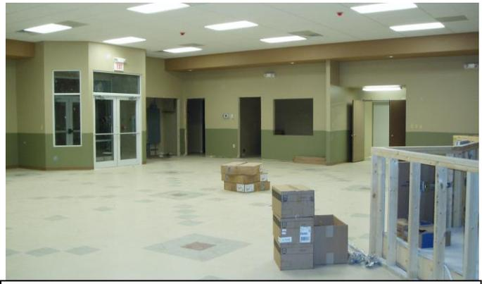
View of the main meeting area, looking at the new entry way and kitchen. The tile flooring is installed and the walls are painted. Exit signs, emergency lighting, and fire detection are also in.
