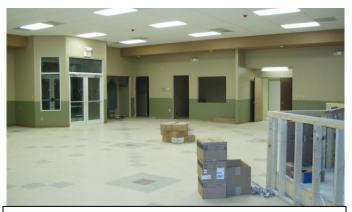
View of the main meeting area, looking at the new entry way and kitchen. The tile flooring is installed and the walls are painted. Exit signs, emergency lighting, and fire detection are also in.
