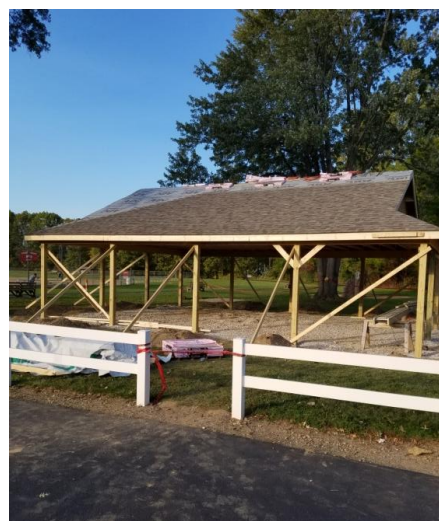
Oct. 9 th – Framing & roof done Shingles started
