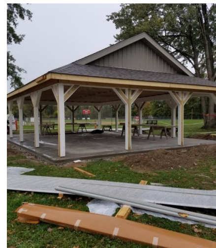
Oct. 15 th – Installation of siding on gables; headers, posts, & angle braces covered with Azek & VersaWrap
