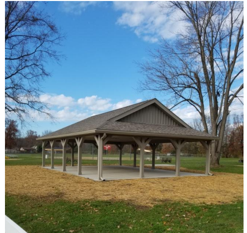
Oct. 23 rd – Gutters installed; Nov. 11 th – Topsoil spread, seeded, and covered
