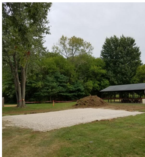
Sept. 30 th – Gravel base constructed
