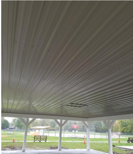
Oct. 19 th – Ribbed, steel barn siding installed on ceiling
