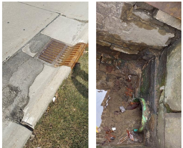
Catch Basin at 6917 Hidden Valley Drive
