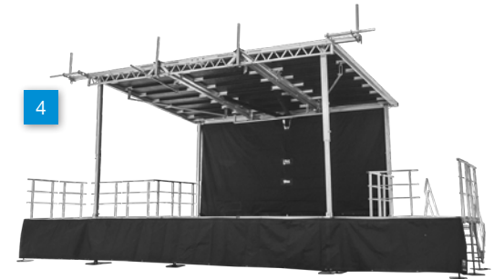
Install stairs, guardrails and add accessories.
