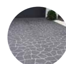
Stenciled concrete driveway
