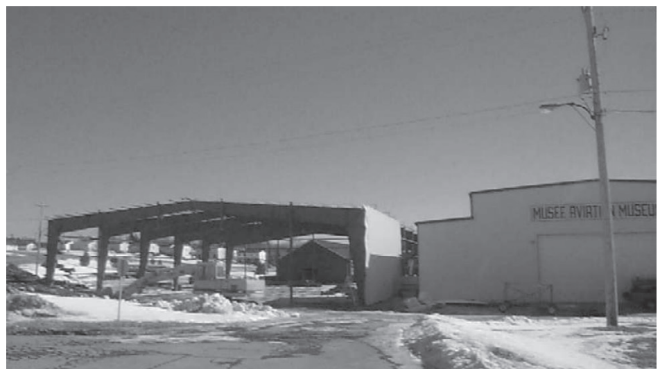
New museum addition from rear of building
