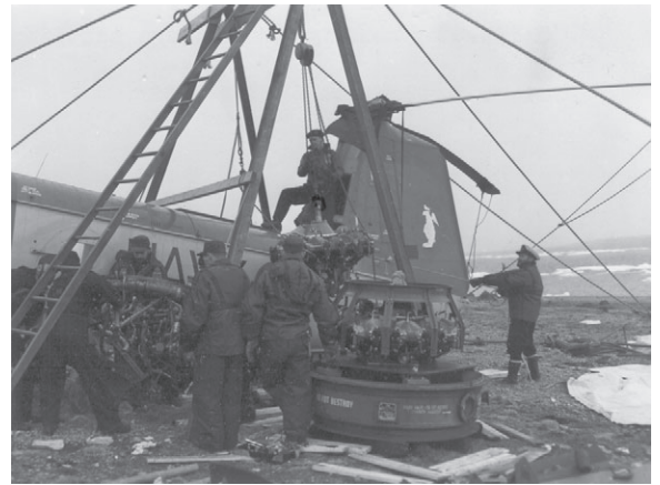
Replacing engine in Piasecki HUP from HMCS Larador at Fort Ross, Bellot Strait, August 1957. (LAB2640)
