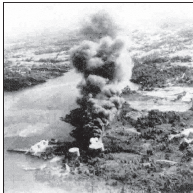
BILL'S ATTACK ON OIL TANK INSTALLATIONS AT DOLVIK
