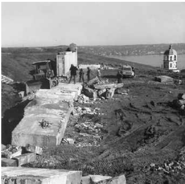
Destruction of Citadel Hill Monument looking NE
