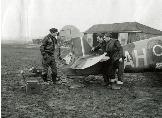
A pilot (left) and two ground crew inspect the flak damage of a 332 (Norwegian) Squadron Spitfire Mk Vb. Close calls like this were commonplace, but flak near the engine, fuel tanks or even the radiator could cause the total destruction of the aircraft. Photo: WarAlbum.ru
