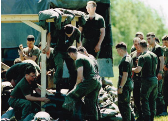
Security of Airfield - building an observation platform
