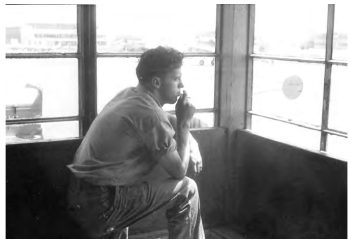
ABAR Guy Lavalee - VU32 'C' Hangar
