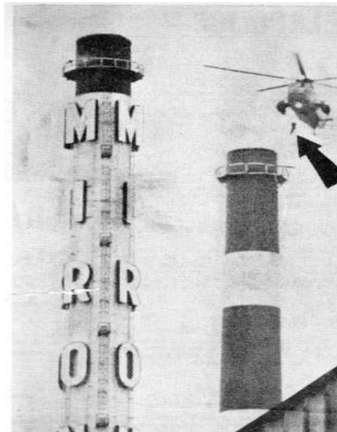
Approaching Grenier on the chimney.
