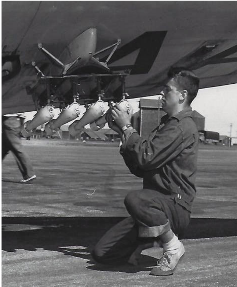
Practice Bombs Being Mounted On Light-Bomb Carrier
