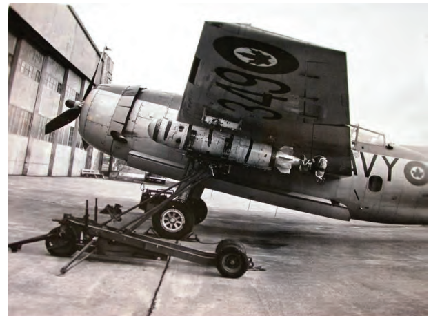
A wing-mounted Mk 43 homing torpedo on NAVY * 349 of VU 33 at Patricia Bay.
