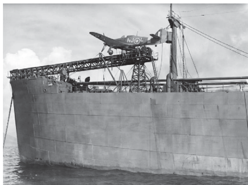
Hurricane Being Mounted on Catapult – Note Wheels Still Down
