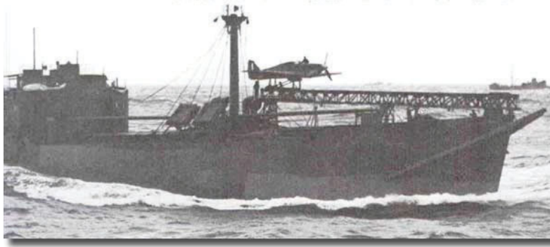
Hurricane mounted on CAM Ship Catapult
