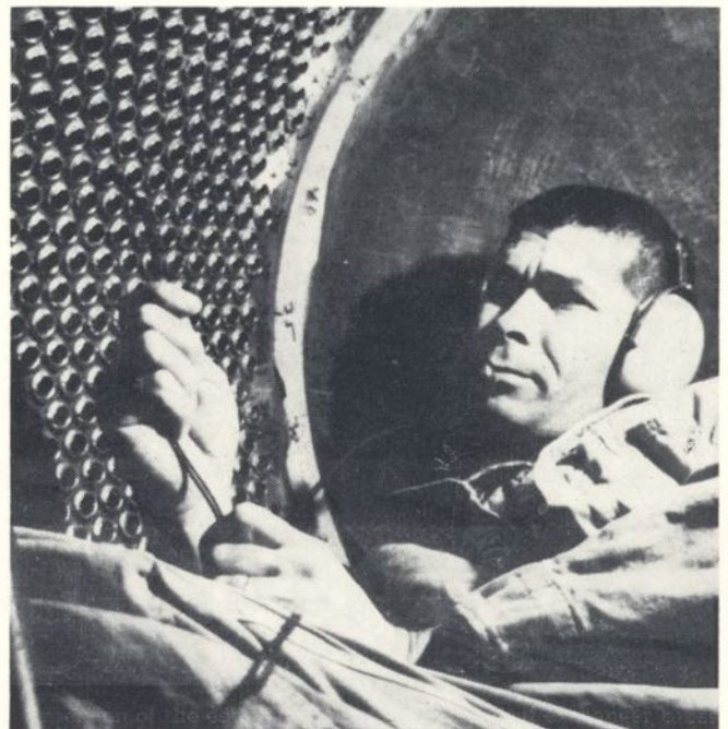
Insertion of the eddy current probe in the heat exchanger tubes in the steam generators required a man to work in a pipe only three feet in diameter. Probe was blown down the tube and withdrawn.
