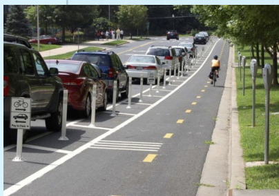
A Protected Bike Lane is a combination of horizontal separation (buffer distance) and vertical separation (e.g. flex posts, bollards, landscaping, curbs, etc.) to protect people bicycling from motor vehicle traffic. The combination of lateral buffer distance and vertical separation elements (such as flexible delineators, curbs or height differences, or vehicle parking) can ameliorate most of the stressors of on-street bicycling while taking advantage of the already paved surface.
