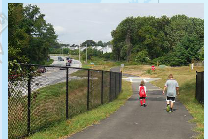
A Shared Use Path is typically a paved off-street trail which provides a high level of safety and comfort for pedestrians and bicyclists of all ages and abilities. To become useful for transportation purposes, shared use paths work best when integrated with an on-street network of bike lanes connecting to key community destinations (schools, libraries, shopping centers, employment areas, etc.)
