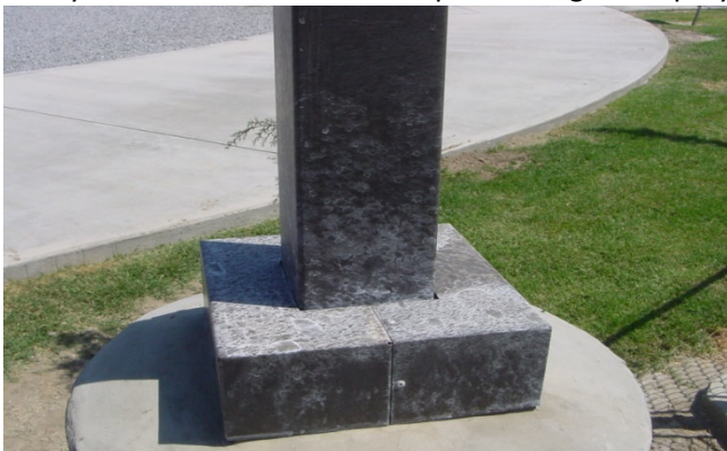
Crusty calcium carbonate build-up from irrigation spray.
