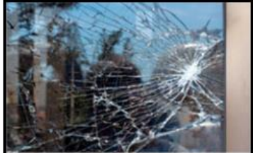
Damage to Property UNDER $5,000
